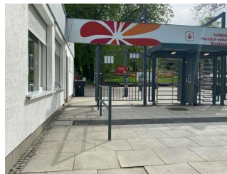
Entrance Gothaer Platz with cash desk
